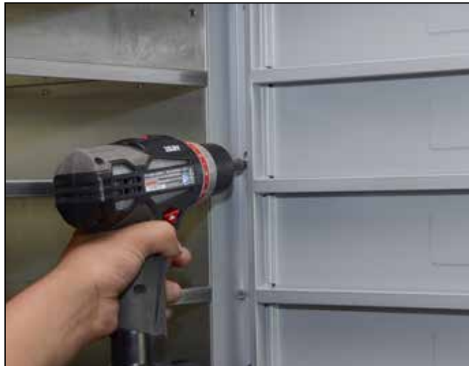
Figure 16– Secure units together using connector machine screws
