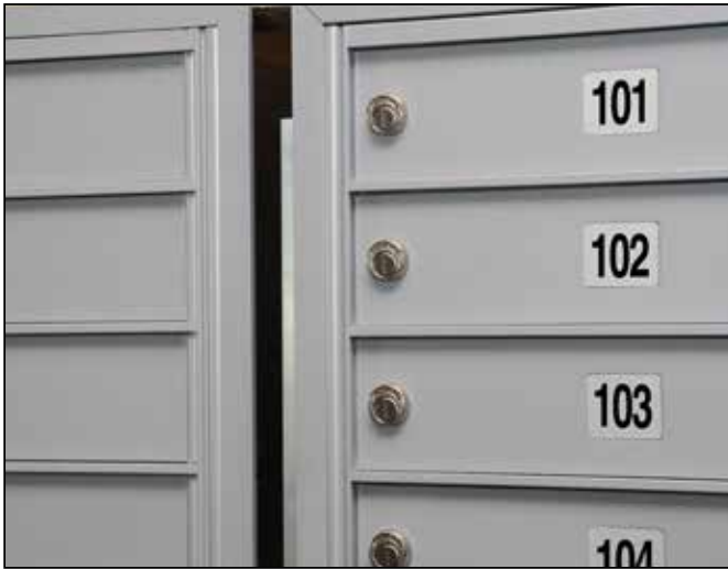
Figure 14 – Align units up next to each other.
