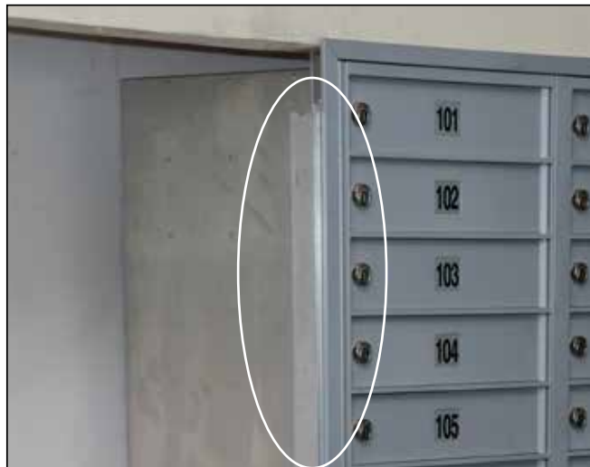
Figure 12 – 4C Connector Bar is now attached to mailbox unit
