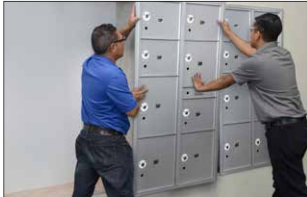
Figure 5C – Butt each unit's trim up against the other.
