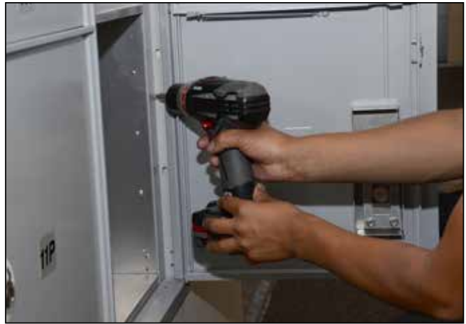
Figure 4 – Bottom side of unit facing wall
