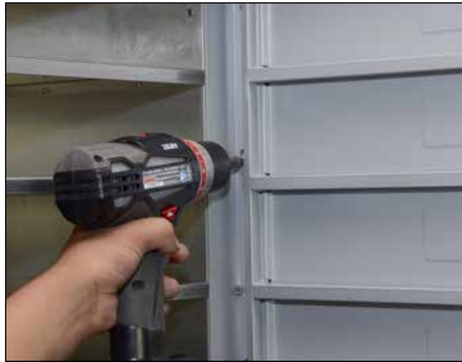
Figure 16– Secure units together using connector machine screws
