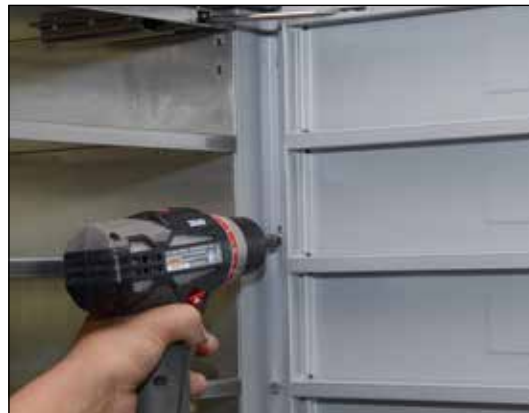
Figure 16– Secure units together using connector machine screws
