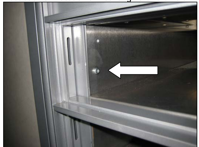
Illustration 3 - Location of Mounting Hardware Hole
