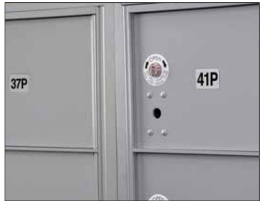
Figure 5C – Butt each unit's trim up against the other.
